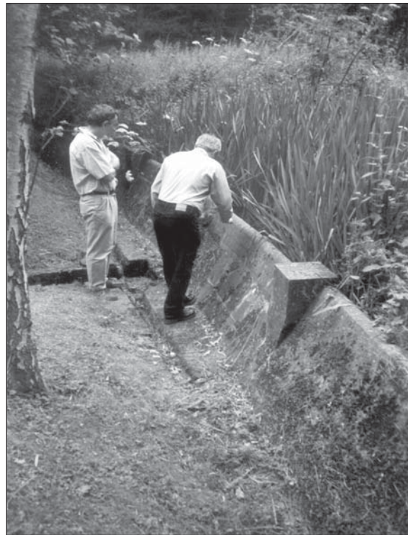
Figure 8. Explosive tests were carried out by the Road Research Laboratory on large-scale models built by the Building Research Station between November 1940 and January 1941.
