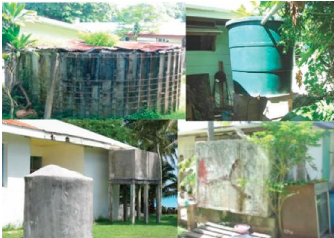
Figure 24: Water infrastructure on Aitutaki. Clockwise from upper left, dilapidated community water tank, household plastic tank, new water tank on community centre, household concrete water tank.
